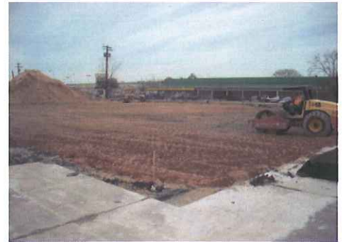
Site - Post Demolition
